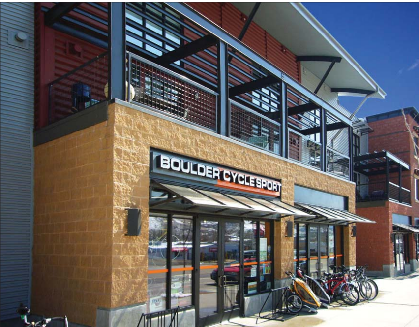
Boulder Mixed-Use Development Boulder, CO
