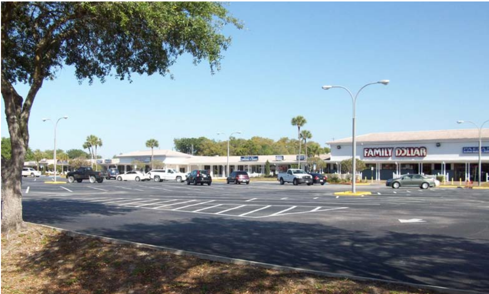
VIEW OF SPRING HILL SHOPPING PLAZA SURFACE PARKING LOT
