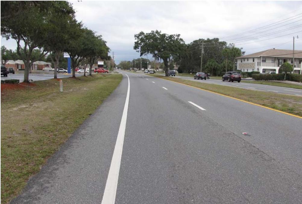
VIEW OF SPRING HILL DRIVE LOOKING EAST
