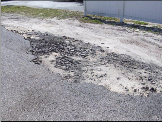
Figure 36. Deteriorating curbs and pavement conditions
