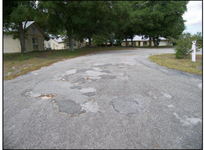
Figure 36. Deteriorating curbs and pavement conditions
