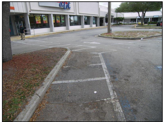
Figure 35. Deteriorating speed humps, pedestrian crossings and disabled parking.
