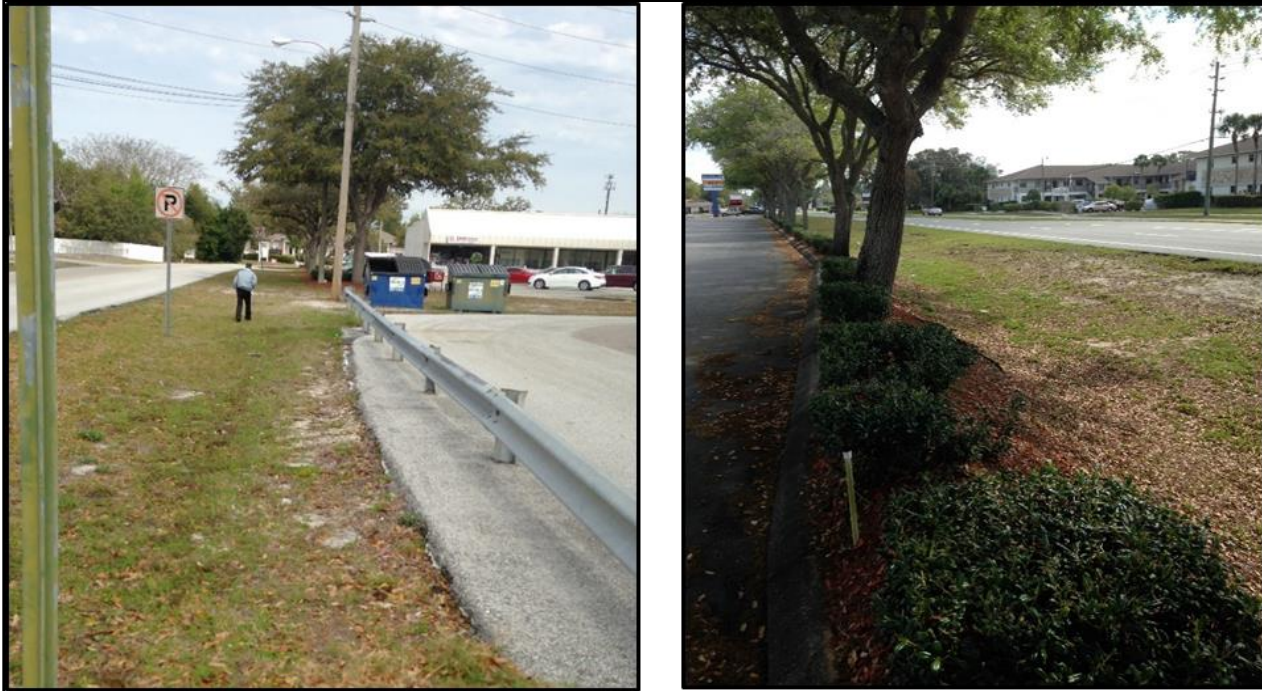
Figure 24: No Sidewalk Access to at Spring Hill Plaza
