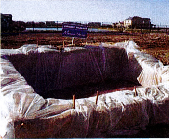
Site built plastic lined pit
