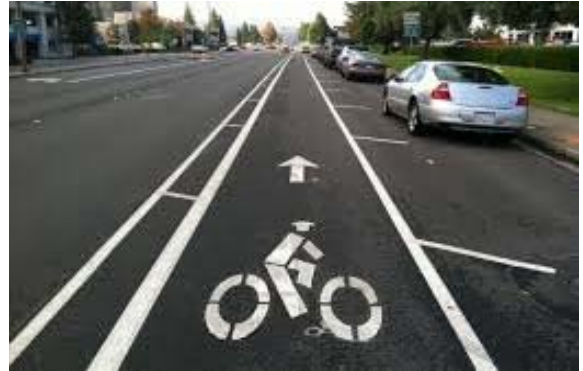
Figure 18: Buffered Bicycle Lane
