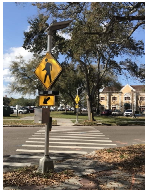
Figure 27: RRFB, St. Petersburg, FL
