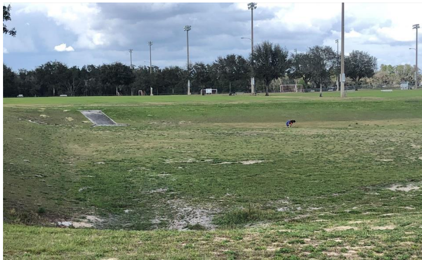
Figure 20: Stormwater Detention Area
