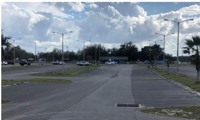
Figure 14: Anderson Snow Park's North Parking Lot
