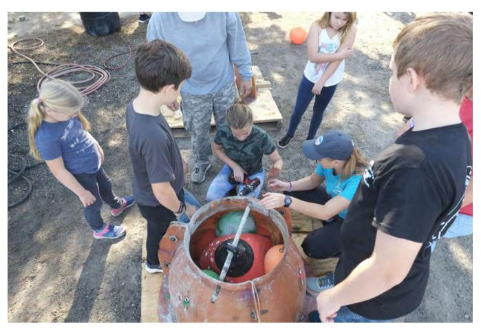
Young members of the SCUBAnauts prepare a concrete mold that will be filled with concrete to create reef domes destined to augment reefs in waters off Hernando County. The rubber balls inside the mold will create voids and entranceways for fish to swim inside.
