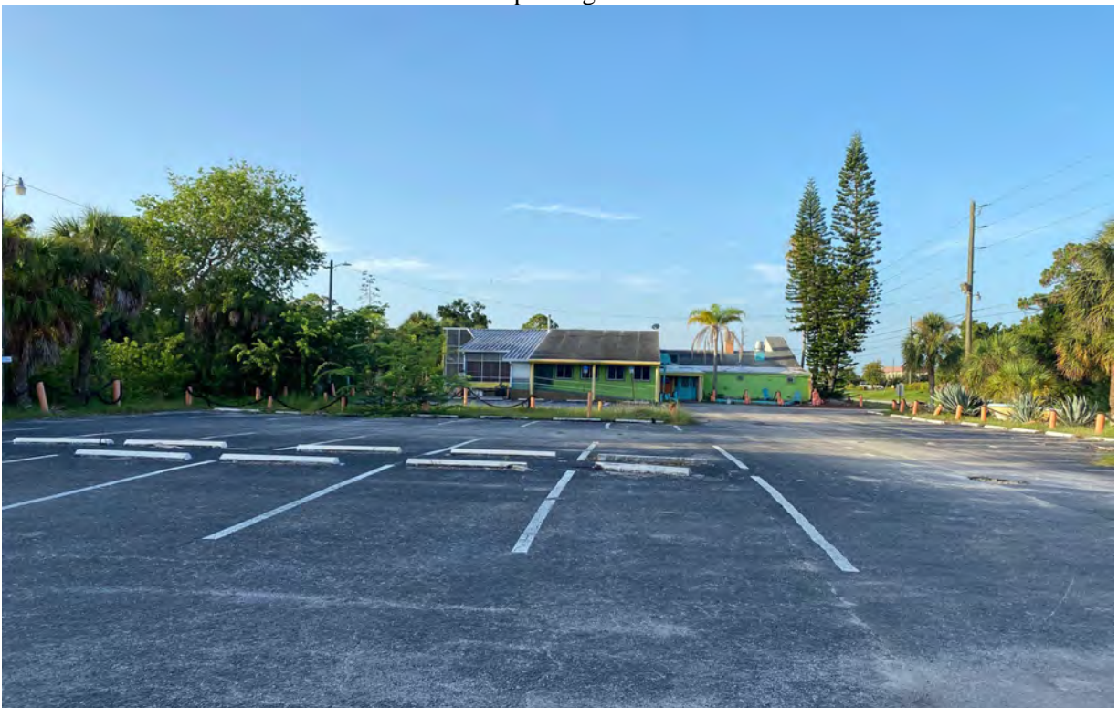
PHOTO 10: Former R Beach Restaurant and parking area.
