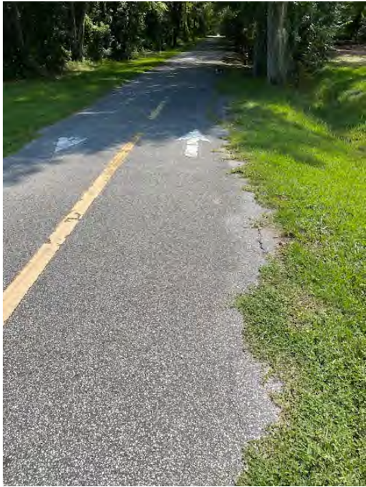
At Jefferson looking east Grass growing over the trail breaking down the edge
