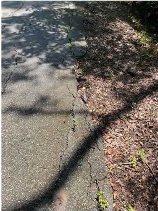
Edge breakdown - typical
