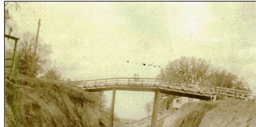
Figure 1-5: Pedestrian bridge used to cross railroad tracks at Hendricks Avenue
