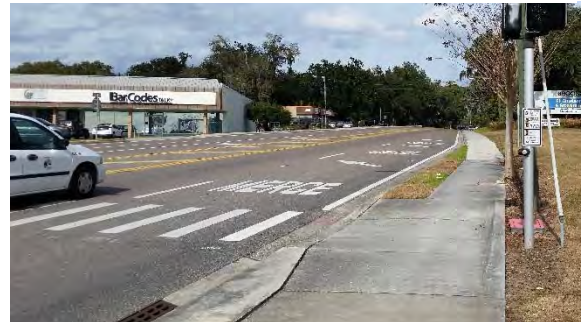
Figure 4: Pedestrian crossing on Broad Street/US-41
